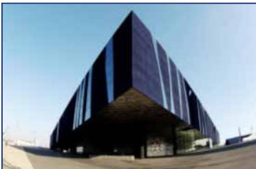
Forum Building Auditorium
